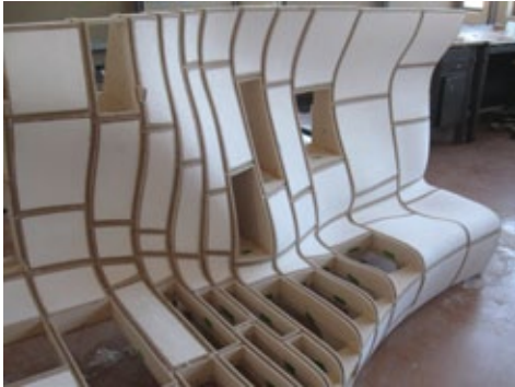
fig.0097 3.8125 installing milled eps panels into panel frames.jpg
