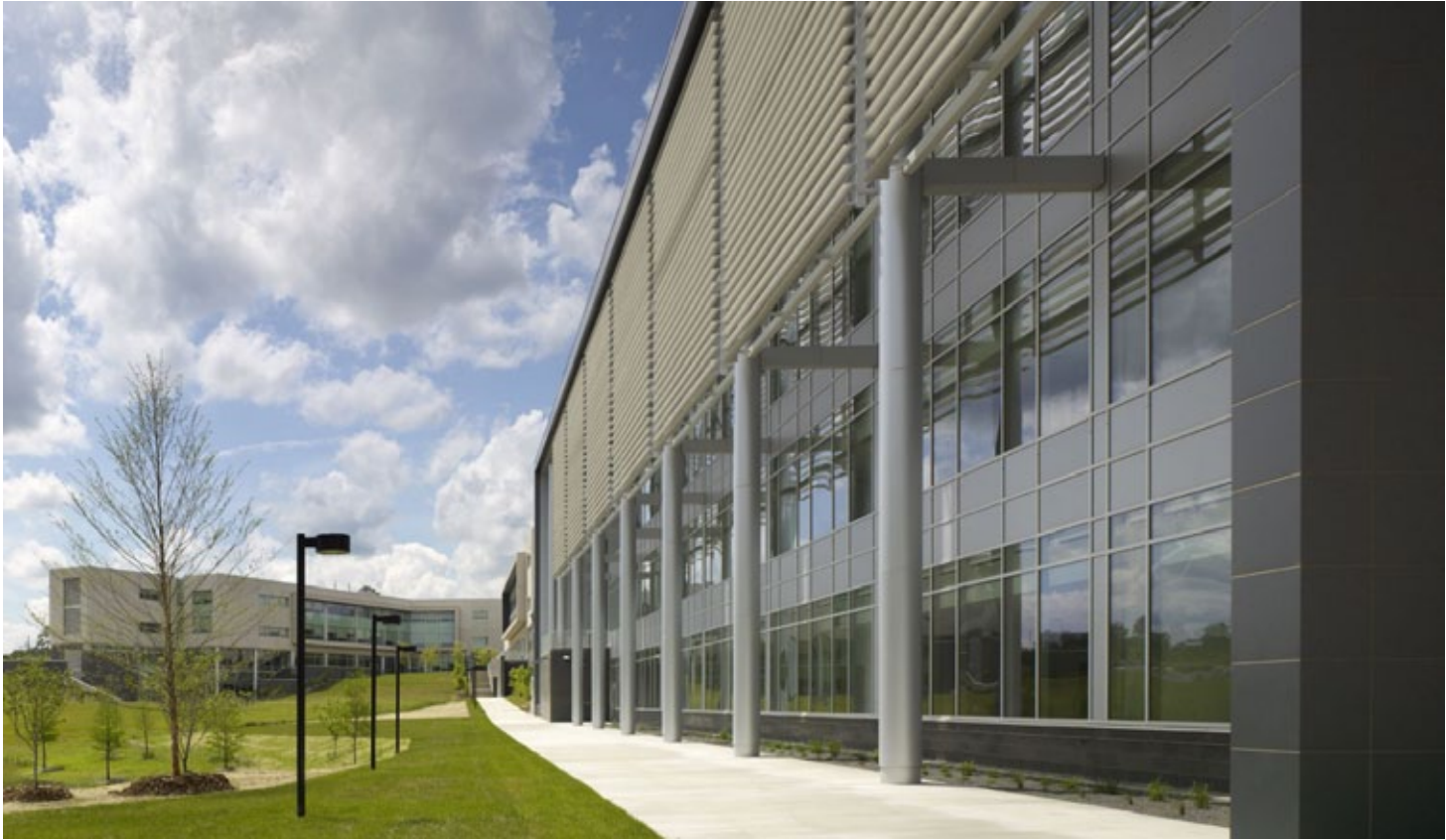
fig.0150 building d south elevation.jpg
