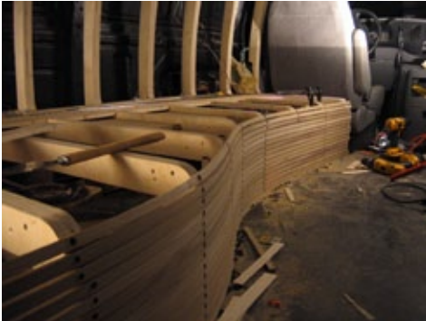
fig.0165 strip planking.jpg
